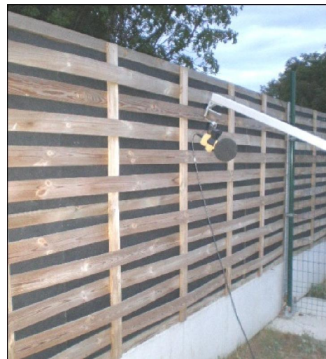
Figure 9. Barrier that doesn't meet minimum dimension requirements.
